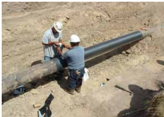
INSTALLING OUTERWRAP
